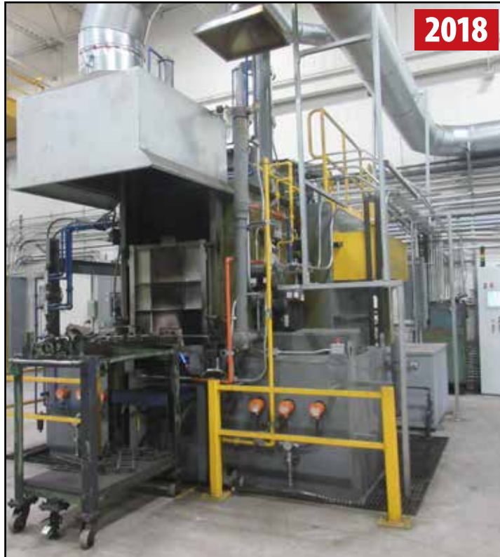
MIDLAND ROSS ALL-CASE 243624 LPG/METHANOL HEAT TREAT FURNACE
